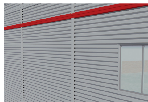
A cap trim is used to cover the end of the sheet while providing a visual break in the horizontal lines.
