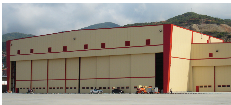
Above: Contrasting cladding emphasizes the sloped exterior wall created by reversing the taper of the columns.
