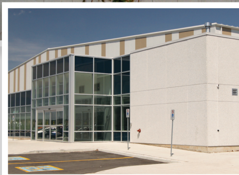
Right: Precast concrete is used in conjunction with insulated metal panels and glass for a custom look.
