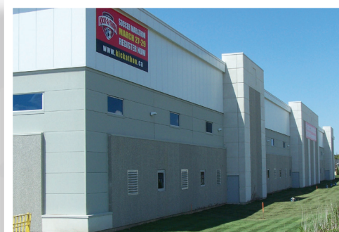
Concrete wall panels are used in conjunction with steel cladding in this soccer complex.
