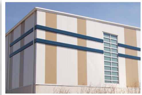
Glass, concrete, and insulated metal panels have been combined on this modern sports facility.
