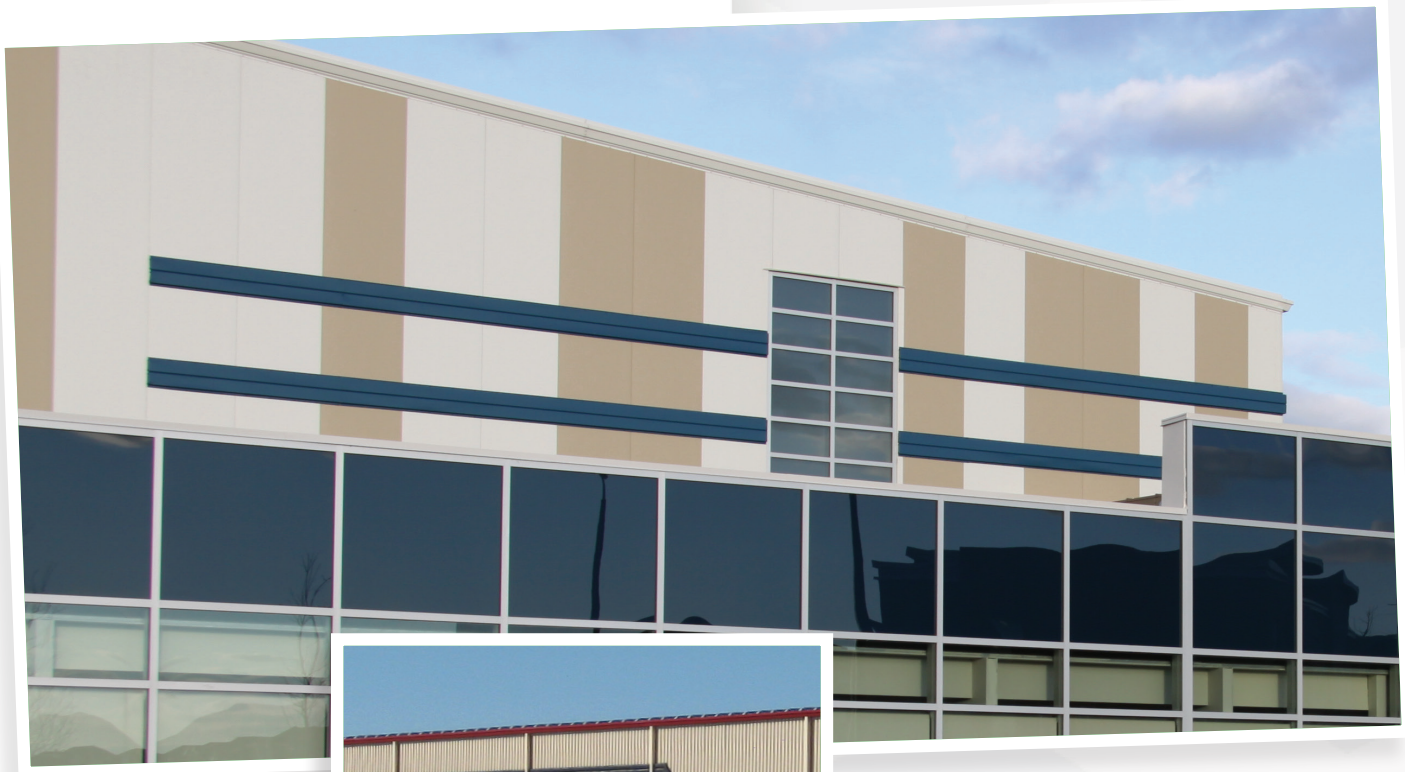
Above: Accent bands fastened to the surface are combined with two different coloured wall panels.
